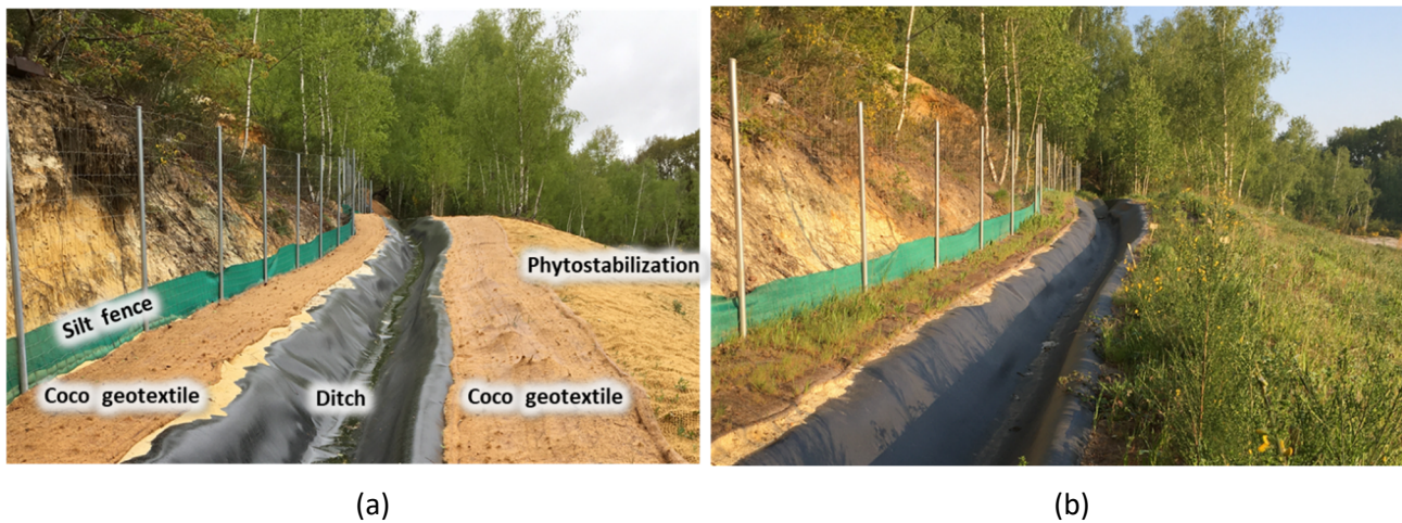
Figure 8 Examples of anti-erosion solutions around upstream rainwater ditches in case study 2: (a) Just after seeding; (b) One year after seeding
